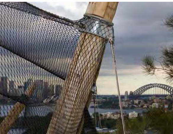
2. Enclosure - blackened stainless steel mesh
