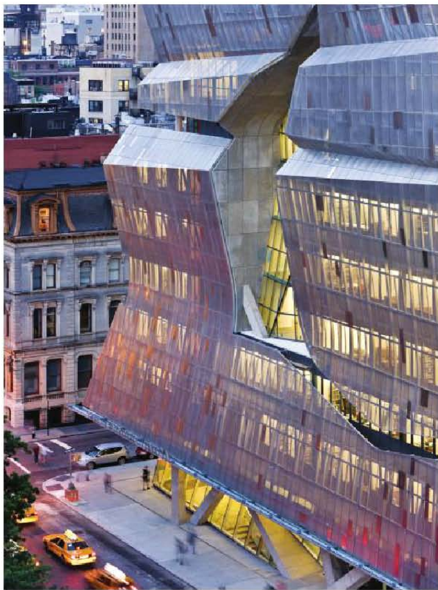
The perforated Type 316 screens around 41 Cooper Square give it a sculptural appearance while reducing its energy consumption.
