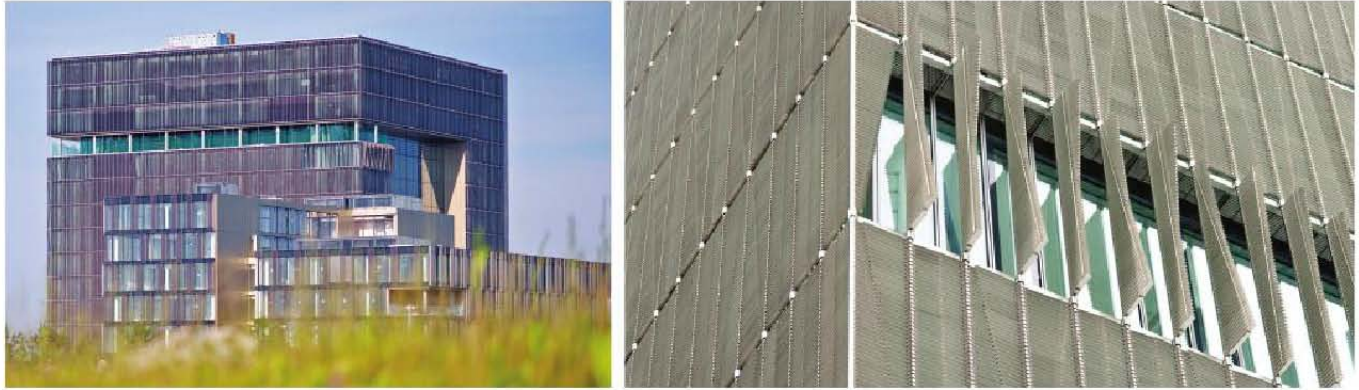
Type 316 stainless steel exterior sunscreens in varying styles were used on this German corporate campus. The systems actively adjust to seasonal and weather conditions in order to reduce energy requirements.
