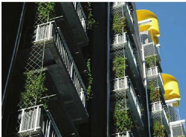
Plant screens were used along the balconies on the north side of Council House No. 2 (CH2) and over the roof deck for shelter from the sun.
