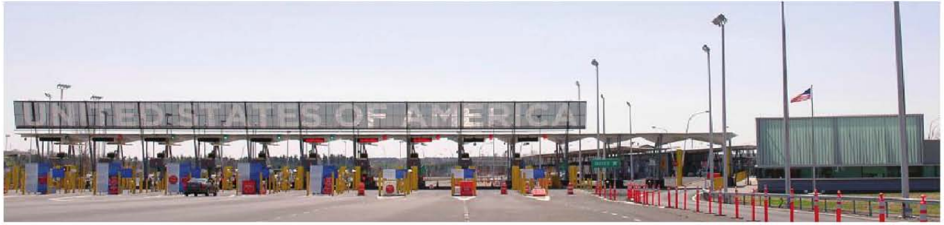
Across from the Québec border, Type 316 woven mesh provides sun shading and improved security for the U.S. Champlain port of entry.
