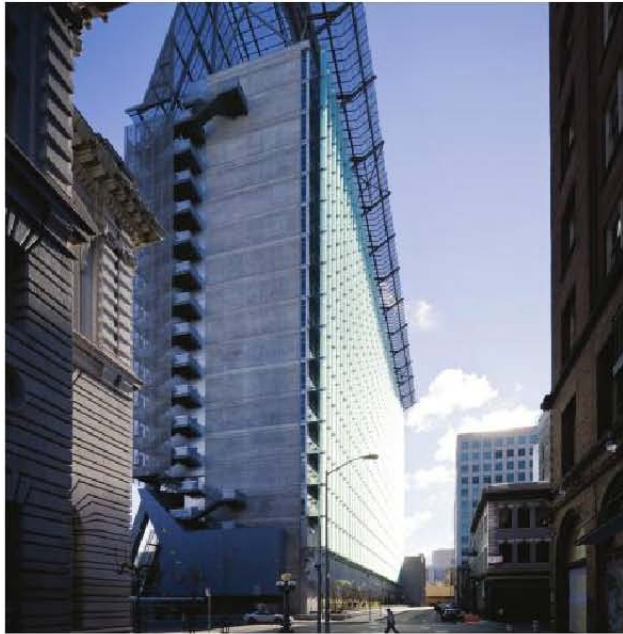
Type 316 perforated screens on the exterior of the San Francisco Federal Building helped eliminate the need for air-conditioning in 70 per cent of the building's occupied spaces and provided a link to the adjoining plaza.
